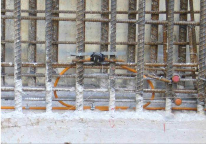
The Normet Injection Tube system is essential for the construction of water tight structures. The joints should be arranged in such a way that crack formation is virtually eliminated.
