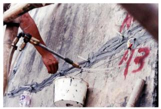
TamRez 310 is a high modulus, high strength epoxy gel designed for the surface sealing of cracks prior to injection, for surface spall repairs and bonding new concrete to old. It is moisture insensitive and will cure in a damp environment.
